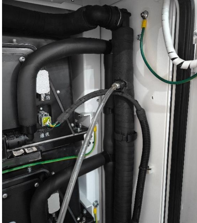
Fig. 9-22 Circulate the coolant carrying free bubbles back into the container
