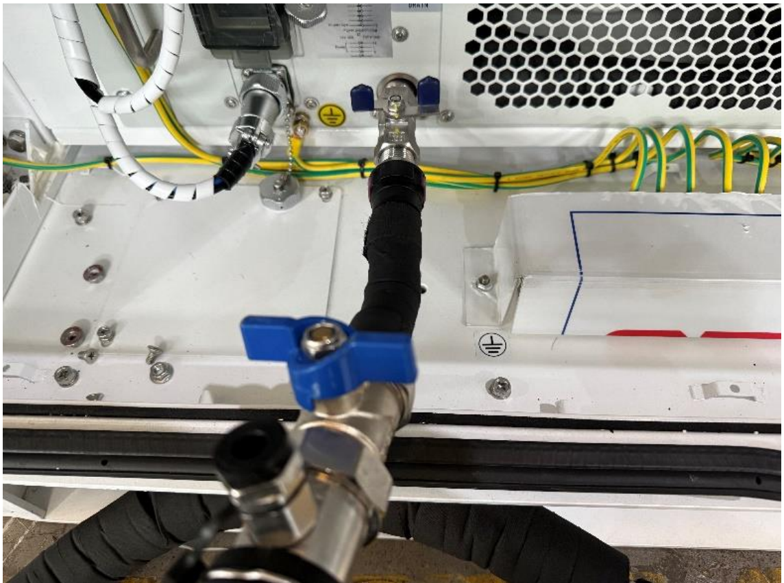
Fig. 9-21 Connect the pipeline of the filling equipment
