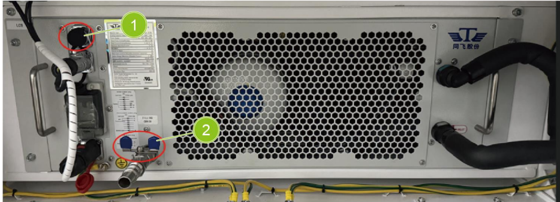
Fig. 9-16 Connect the quick plug and close the drain valve
