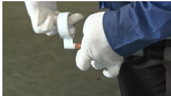
Figura 3-19 Envolver el conductor
